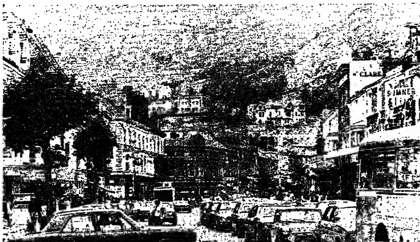
One of Llandudno's main shopping thoroughfares, Mostyn Street. A study recommends restoration of the cast iron verandas over the shops, a distinctive feature of the resort's Victorian traditions.
